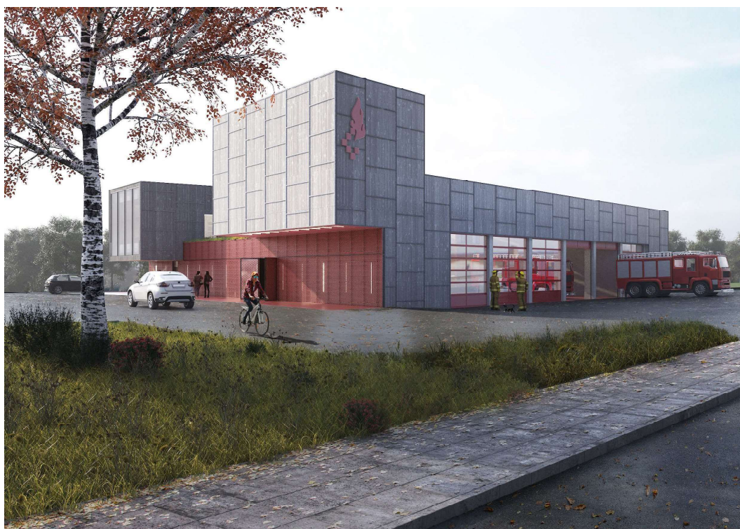
Ny brandstation i Lisbjerg – Station Aarhus Nord
